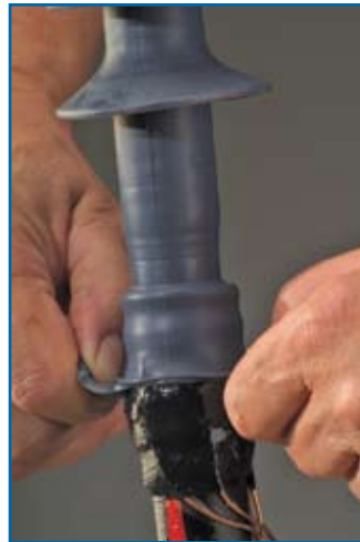
Step 10. Fold down the skirt over the mastic to seal the cable entrance.
