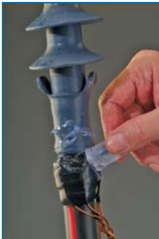
Step 9. Apply silicone lubricant to skirt and mastic area.
