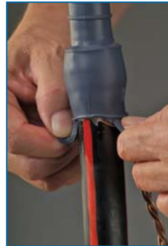
Step 10. Fold down the skirt over the mastic to seal the cable entrance.
