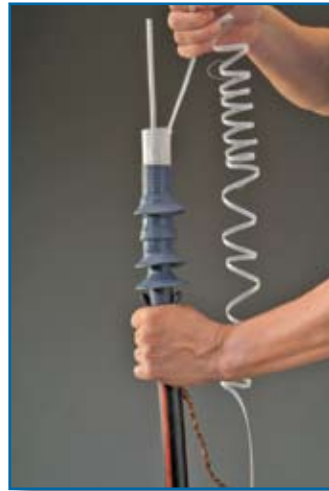
Step 8. Shrink into place by unwinding the removable core.
